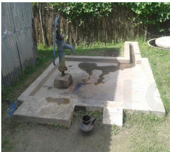
Figure 23: Cemented sanitary Tube-well
